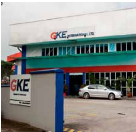
Warehouse at Jalan Besut
